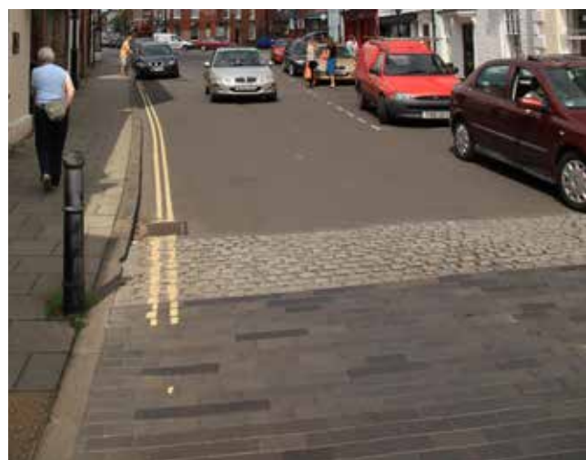
Change in carriageway material at pedestrian crossing
